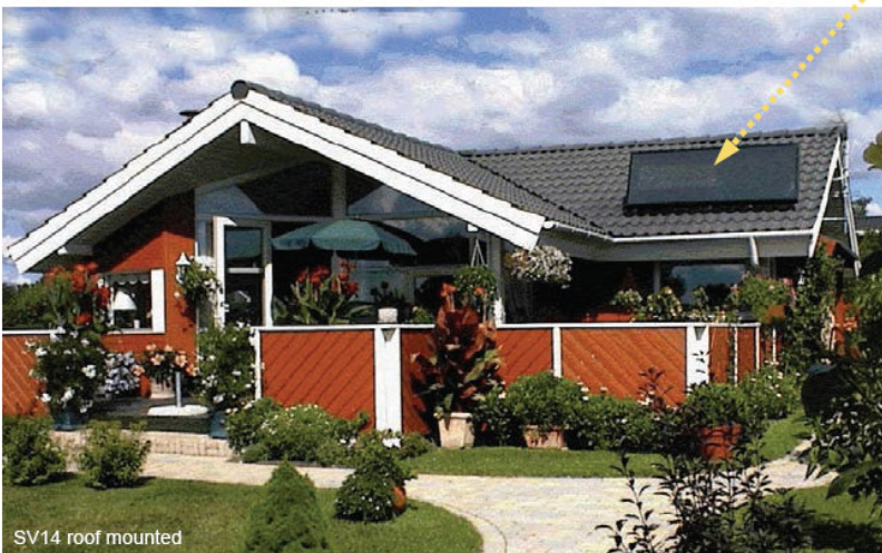
SV14 roof mounted
